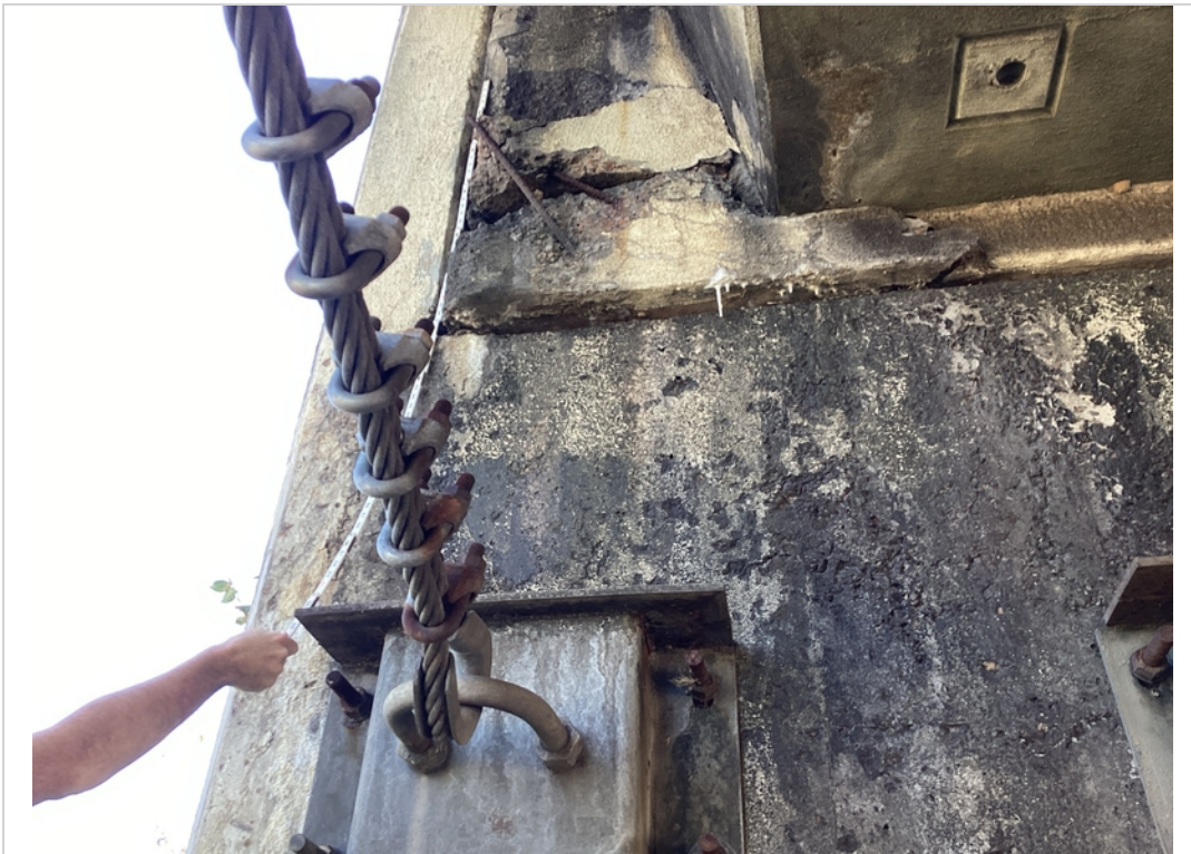
Spall steel back wall span 1
