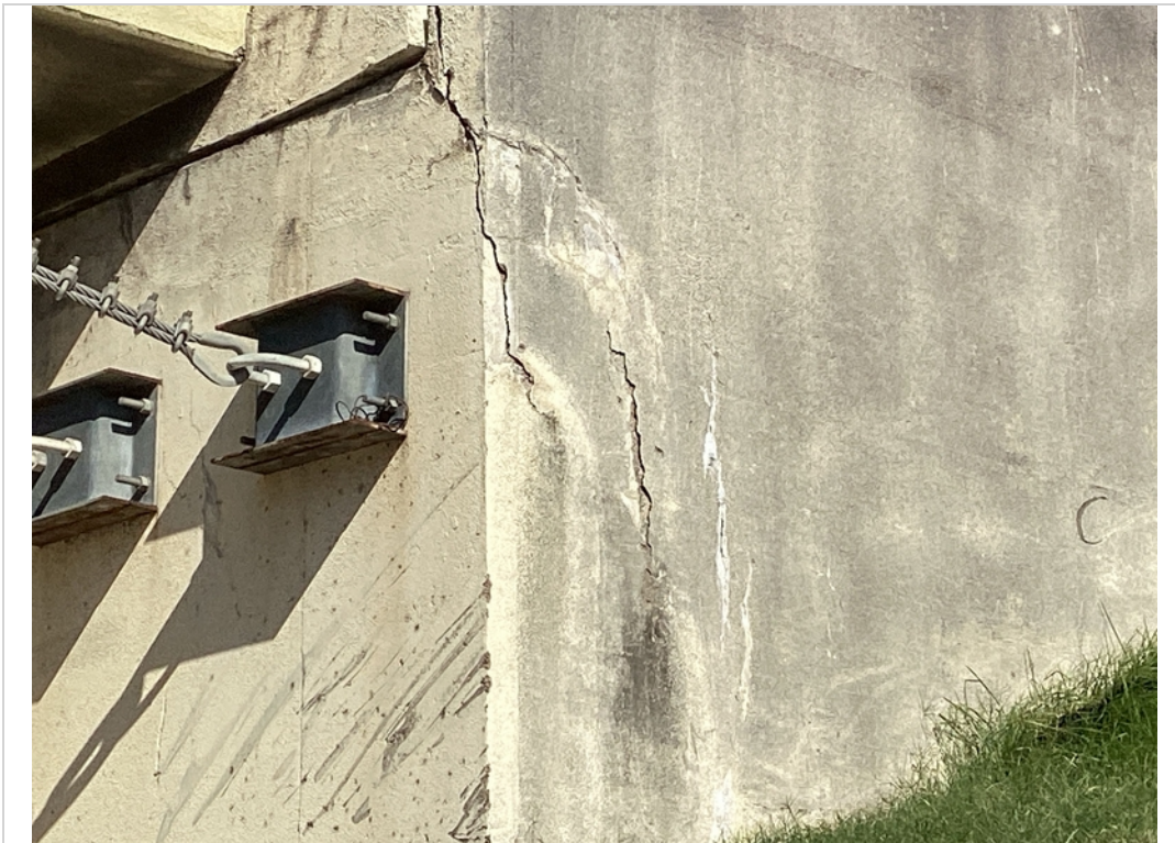
Abutment 2 impending spall
