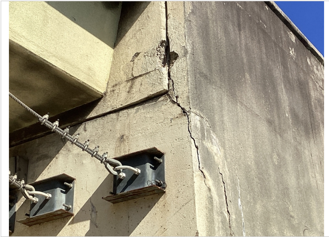
Abutment 2 spall
