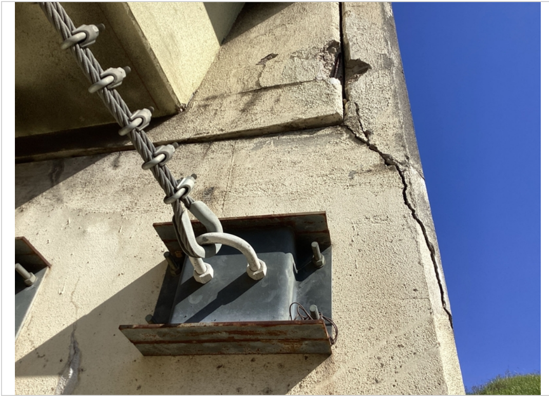
Spall steel back wall span 1
