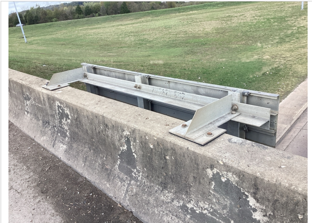
Bridge mounted sign upper connection
